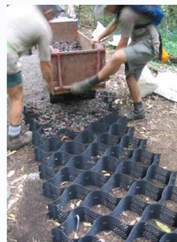
Figure 8. Track construction using large-cell perforated plastic moulds at a site that is muddy for part of the year. The cells are filled with mixed bark and gravel and the structure is then capped with gravel to allow water movement and root development in the cells.
